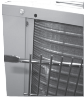
Fig. 2 - Removing Outdoor Grill
