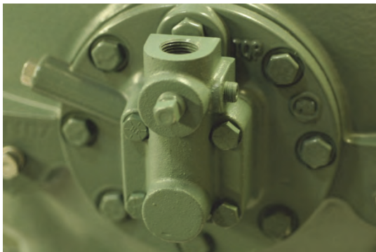
Fig. 19 — OPSS Sensor Block Installed
