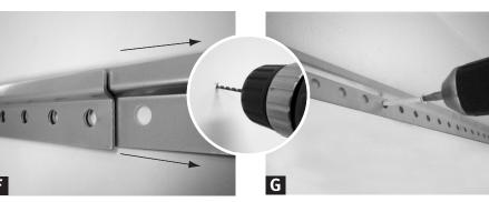
Secure second rail from right side Install screws into studs (or anchors) along rails. Secure rail in all studs.
