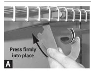
Install rod hanger Install rod hanger into bottom of bracket by tilting it backward until it locks in place. Note: be sure to press rod hangers firmly into place for proper installation.
