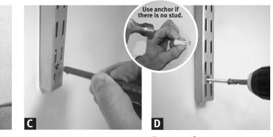
Secure Mark bottom hole of each upright. Drill 1/8" pilot hole into stud. (Use wall anchor and 3/8" bit if there is no stud.)
