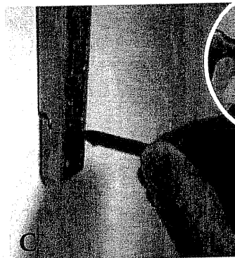
Mark bottom hole of Upright. Drill 1/8" pilot hole into stud. (Use Wall Anchor and 3/8" bit if there is no stud.)
