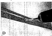
Starting at left side, fasten the FIRST TWO screws into studs (or anchors). Do not fasten remaining screws until after next step.
