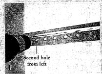
Mark and drill a 3/8" hole (for a Wall Anchor) in the second Hang Rail hole from the left.
