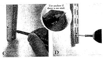
Mark bottom hole of each Upright. Drill 1/8" pilot hole into stud. (Use Wall Anchor and 3/8" bit if there is no stud.)
