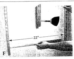
Hang another 47.5" Upright on the Rail and use one of the 22" Rail Covers to space over 22". Drill 1/8" pilot hole and fasten screws in bottom hole. (Use Wall Anchor and 3/8" bit if there is no stud.) Place 22" Rail Cover over Rail between Uprights. Repeat Step F for one or two more Uprights (if space allows).
