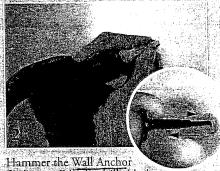
Hammer the Wall Anchor flush to wall in the drilled hole. Insert Anchor Key to engage Anchor.
