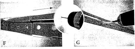
Slide second Hang Rail to the right wall of the closet, and then back it away from the right wall until the holes in the two Rails line up. Repeat Step C to secure to the wall.
