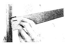
Insert Brackets into Uprights at desired locations. Note: Install Brackets and shelving at the top first and work down. Brackets will not fit into upper two slots of each Upright.
