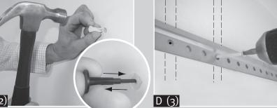
Drywall anchor installation\* Mark and drill a 3/8" hole (for a wall anchor) in the second hang rail hole from the left. To compress the anchor, fold the sides and bend. Hammer the wall anchor flush to wall in the drilled hole. Insert anchor push pin to engage anchor.
