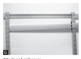
Attach 22" rail cover If the space between the last uprights is less than 22", you may choose to cut rail cover with scissors to fit. Note: Add-on accessories require uprights to be
