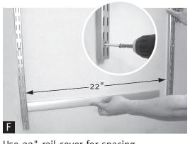
Use 22" rail cover for spacing Hang another 47.5" upright on the rail and use one of the 22" rail covers to space over 22". Drill 1/8" pilot hole and fasten screws in bottom hole. (Use wall anchor and 3/8" bit if there is no stud.) Place 22" rail cover over rail between uprights. Repeat step F for additional upright (If space allows).
