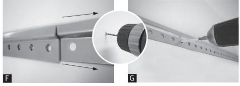
Extend second hang rail Slide second hang rail as far right to the wall as possible while still maintaining hole alignment. Repeat step C to secure to the wall. If there is not a stud within 4" of the RIGHT end of the hang rail, repeat the dry wall anchor installation
