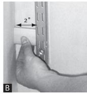
Position at 2" Position both outside uprights 2" from the right and left corners by using the 2" rail cover for spacing.
