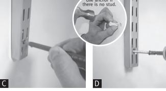
Secure Mark bottom hole of each upright. Drill 1/8" pilot hole into stud. (Use wall anchor and 3/8" bit if there is no stud.)
