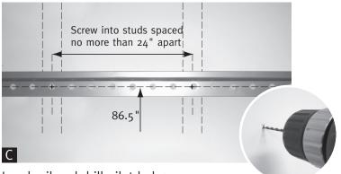
Level rail and drill pilot holes Level hang rail and mark holes 86.5" above floor that land on studs, then drill 1/8" pilot holes for screws.
