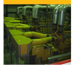
Four specially designed Cat® 3616 generator sets run on crude oil to provide a reliable source of power and heat to the Polyus gold mine and the surrounding community.
