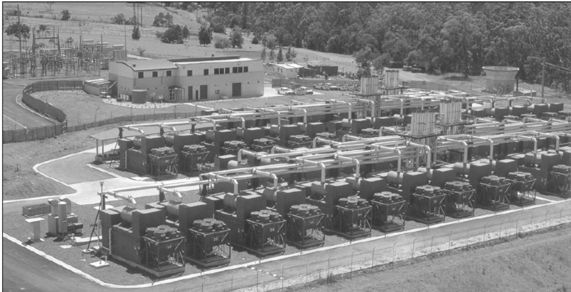
Figure 12: Appin and Tower Coal Seam Energy Project
