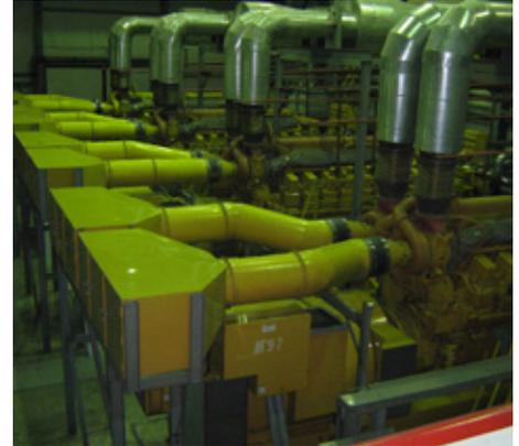
*Four specially designed Cat® 3616 generator sets run on crude oil to provide a reliable source of power and heat to the Polyus gold mine and the surrounding community.*
