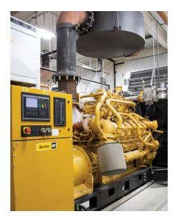
The reclamation facility is now served by an on-site power plant equipped with four Cat<sup>®</sup> G3512 gas generator sets, resulting in higher reliability and the ability to lower energy costs by peak shaving.
