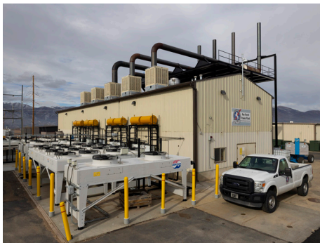
In 2002, Heber Light & Power became one of the first public utilities in the world to install Caterpillar's line of advanced gas-fueled generator sets.
