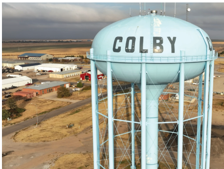
Colby, Kansas has operated a municipal power plant since 1910. Recent growth prompted city management to replace outdated power systems with new Cat® C175 gensets.
