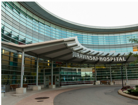
Juravinski Hospital is one of seven hospitals in the Hamilton Health Sciences (HHS) network, which serves a population of 2.3 million in the province of Ontario.
