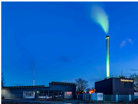
Stadtwerke Lemgo, a local municipal utility, is reducing the impact of its operations by using combined heat and power (CHP) system powered by Cat natural-gas generator sets, a solar thermal system, and a heat pump using water from the Bega River.
