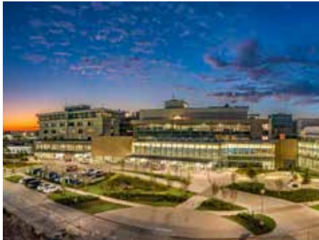
Children's Hospital New Orleans switched over to its Cat® diesel generator sets before Hurricane Ida made landfall to avoid any potential power interruptions to surgeries or hospital services.
