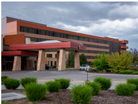
The Shoshone-Bannock Casino Hotel in Fort Hall, Idaho, depends on standby power from permanent Cat® 3516 and C175 diesel generators and uses Cat XQ125 mobile generators to power outdoor events.
