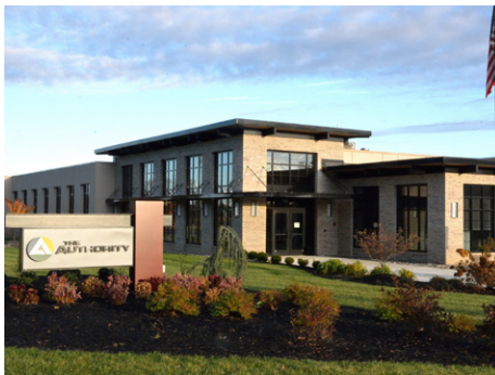
The Authority is the only landfill operator in New Jersey to operate a microgrid, maintaining and operating its own electrical infrastructure.
