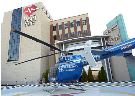
Emergency power is critical for St. Luke's, which has 16 operating rooms that are fully utilized from 12 to 16 hours daily.
