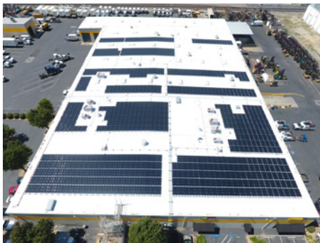
Holt of California sought to further reduce its carbon footprint by opting to install two solar arrays with a combined total output of 825 kW.
