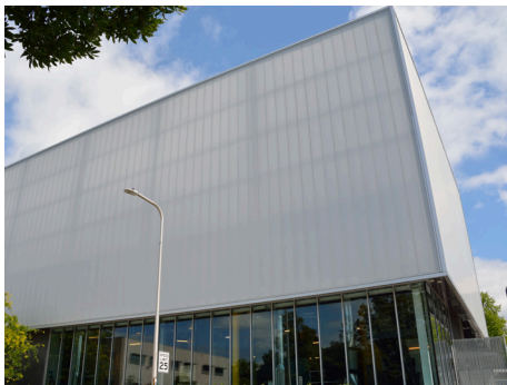
The Campus Energy, Utilities and Operations (CEUO) department is responsible for providing uninterruptible and reliable emergency power and chilled water to all UW facilities.
