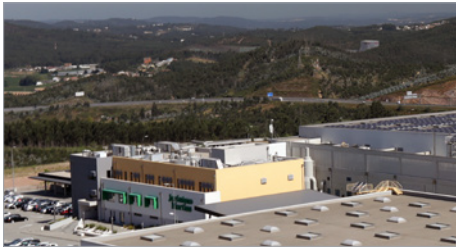
Jerónimo Martins is the biggest food distribution company in Portugal and supplies more than 483 of its own supermarkets across the country through 11 distribution centers.
