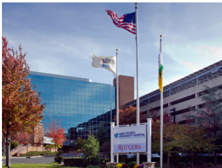
In 2011, Saint Peter's embarked on an energy-savings initiative that included a comprehensive upgrade of the hospital's electrical systems.
