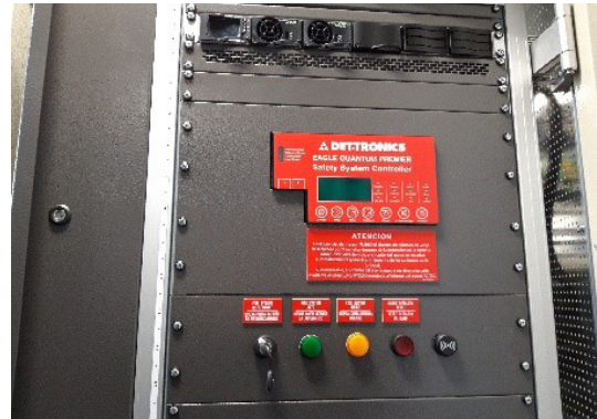
EQP Controller Installation
