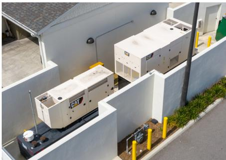
*The standby power solution for HarborChase of Wildwood includes sound-attenuated enclosures, integrated diesel fuel storage and automatic transfer switches.*
