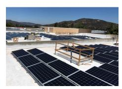
A 492 kW solar array was installed on the roof in the summer of 2020, featuring 1,348 Cat® PVC solar modules, each providing 365 watts of power.
