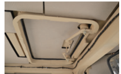
Emergency egress hatch.
