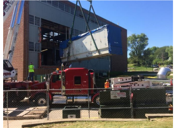
Installing Taurus 70 – Central Heating Plant (Source: Eastern Michigan Univ.)
