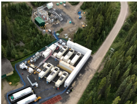
An important stage of AltaLink's project involved replacing the structures and conductor in the mountainous terrain, which did not allow for the construction of a temporary line to keep the lights on for the loads west of Banff.
