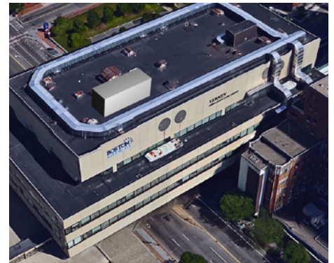
The cogeneration system supplies reliable power to the 514-bed hospital independent from the grid during a power outage.
