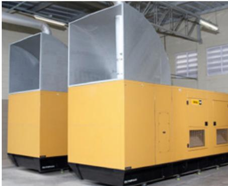
*Liotécnica uses two Olympian™ diesel generator sets for a constant flow of power when the prime utility source fails and for peak load shaving.*
