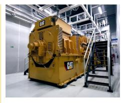
The cogeneration plant has two Cat® CG260-16 gensets that produce a total of 8 MW of electric power and one absorption chiller, which produces 988 tons of chilled water for air conditioning.
