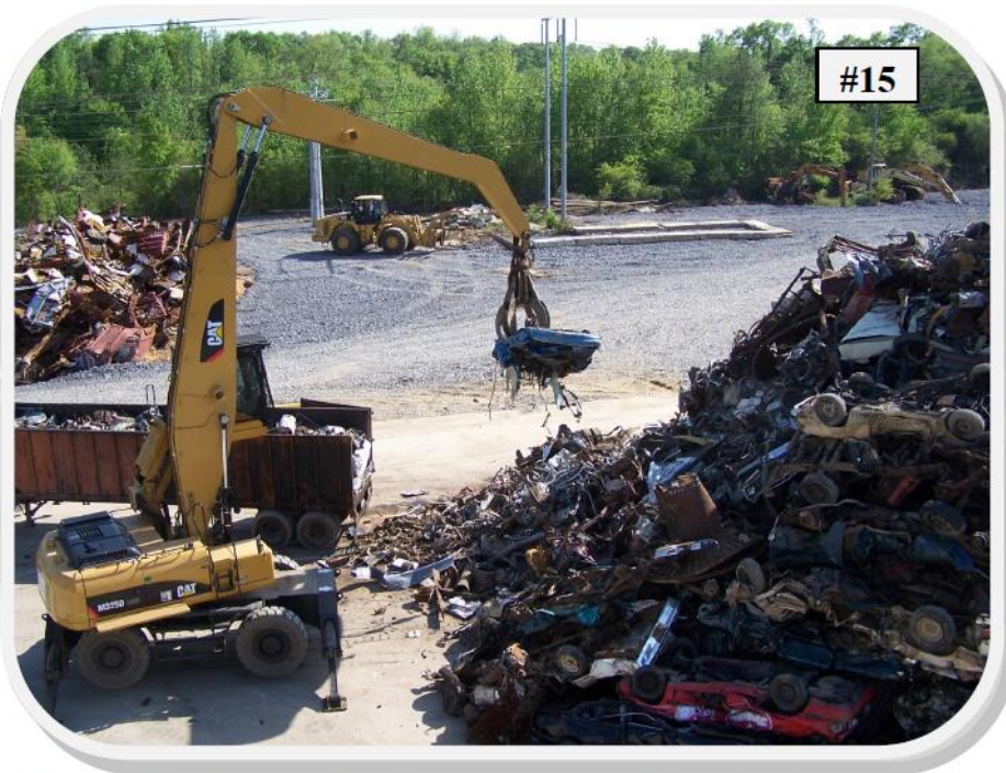
The M325D Material Handler picks up scrap to load the semi trailer.
