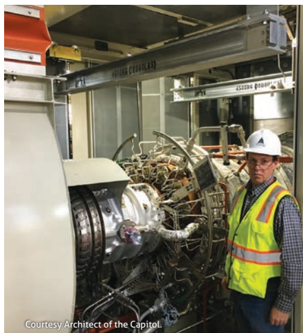
AOC engineer with the newly installed combustion turbine.
