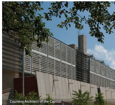
The West Refrigeration Plant.
