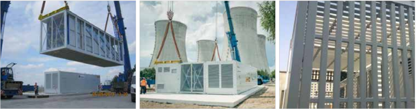
Figure 1: Modular Emergency Power Source
