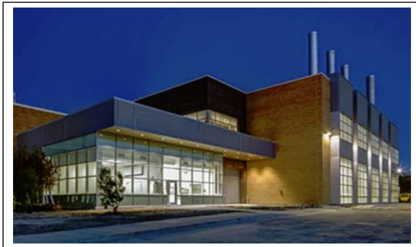
New Central Energy Facility with 5.7 MW Gas Turbine CHP System
