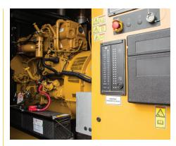
The Crossfield mushroom farm has two large boilers and a chiller, which the C18 generator backs up along with the rest of the farm's electrical load.
