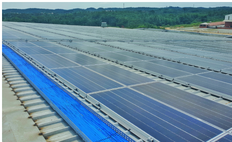
The hybrid energy solution at Mantrac's component rebuild center in Takoradi, Ghana, includes 1,290 rooftop-mounted Cat® photovoltaic modules.
