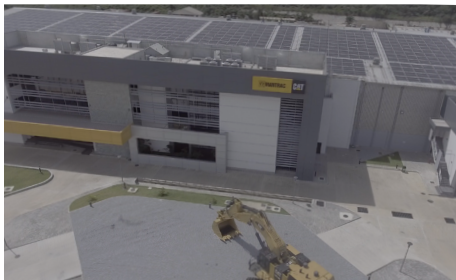
The Mantrac component rebuild center in Takoradi, Ghana, is outfitted with the latest technology to restore like-new performance of Cat® machinery.
