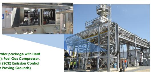
7.9 MW Combustion Turbine Generator package with Heat Recovery Steam Generator (HRSG); Fuel Gas Compressor, and Selective Catalytic Reduction (SCR) Emission Control (photo courtesy of Aberdeen Proving Grounds)
