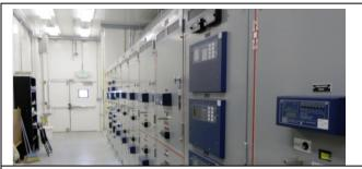
New switchgear installed at the central power plant. This switchgear allows the CHP project to meet critical loads when switching to island mode operation.
