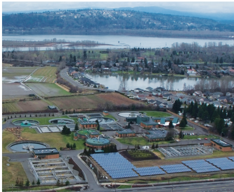
Cat® generator sets help the Gresham Wastewater Plant achieve energy net zero.
