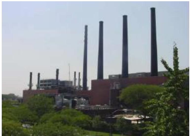
UIC West Campus CHP Facility
