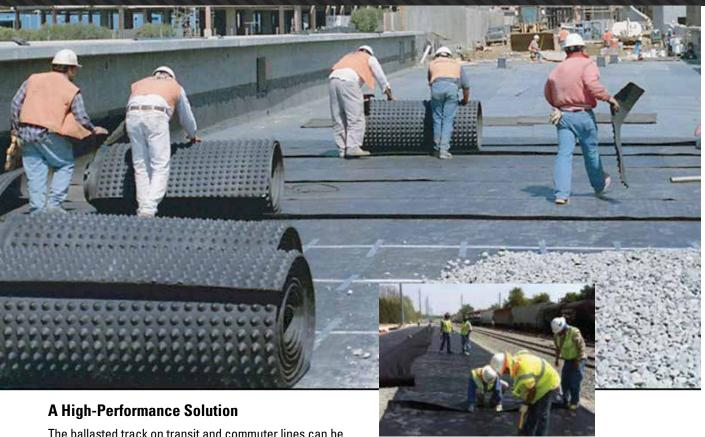
Limits structure-borne vibration, reduces impacts and cuts tamping by 70%.
