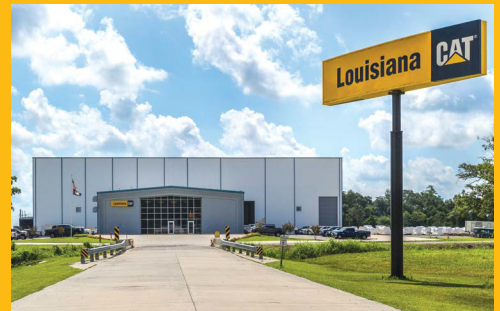
Louisiana Cat's New Iberia facility is the dealer's energy and transportation headquarters.
