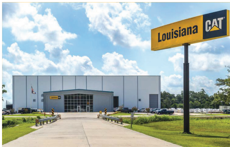
The Louisiana Cat New Iberia facility is the dealer's energy and transportation headquarters.
