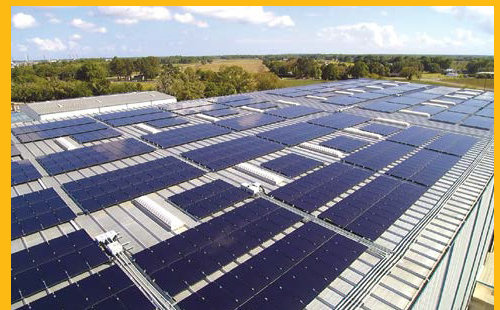
Louisiana Cat installed 1,550 Cat® PVT115 photovoltaic solar panels atop its service building.
