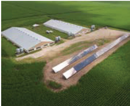
Sitruc Pork operates six hog sites near Waverly, Iowa, U.S.A. One site installed more than 800 Cat® solar panels to help offset utility costs.
