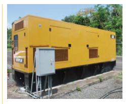
A Cat® 500 kW 3456 enclosed diesel generator set was installed in 2008. In four years, the machine only has accumulated 900 hours, which is mainly due to weekly routine maintenance tests.
