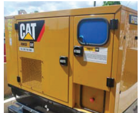
A Cat® 20 kW D20-6S diesel generator set was chosen to provide power when service from the utility is interrupted.
