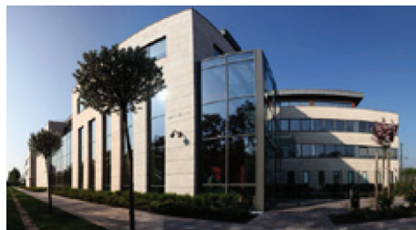
Located in Budapest, Hungary, DoclerWeb provides co-location, server hosting and application hosting to hundreds of customers.
