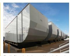
The i/o Phoenix site is served by a dedicated, on-site substation expandable to 120 MW. Empire Power Systems has deployed and supports more than 27 MW of uninterruptible power supply (UPS) systems and 58 MW of Cat® 3516 back-up generators that feed into paralleling Cat switchgear.
