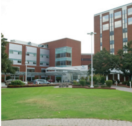
After witnessing the devastation of Hurricane Katrina, the facility management team at Cape Fear Valley Medical Center re-evaluated their emergency power capabilities.
