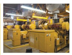
Four Cat<sup>®</sup> 3512 diesel generator sets serve as emergency backup power for the life-safety systems and other operations of three hospitals and smaller facilities, ensuring a continuous supply of power.
